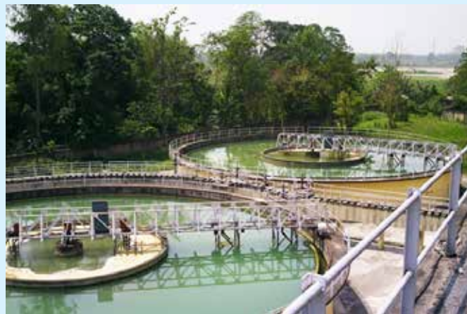
CLARIFLOCCULATOR TANKS
