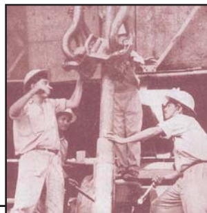
EXPLORATION FOR OIL : Drilling crew preparing to pick up a string of drill collars.
